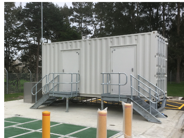
TYPICAL CONTAINER INSTALLATION FOR A PUMP STATION
